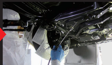
Spray "Brown" to the hollow & cutout areas through the existing hole (approx. 0.75 - 1 ℓ)
